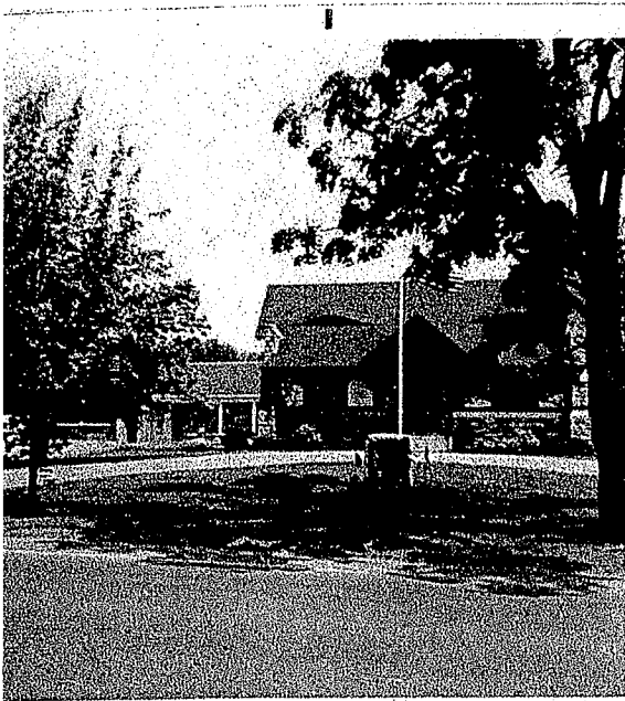
3 June 1973 - Progress on Library
